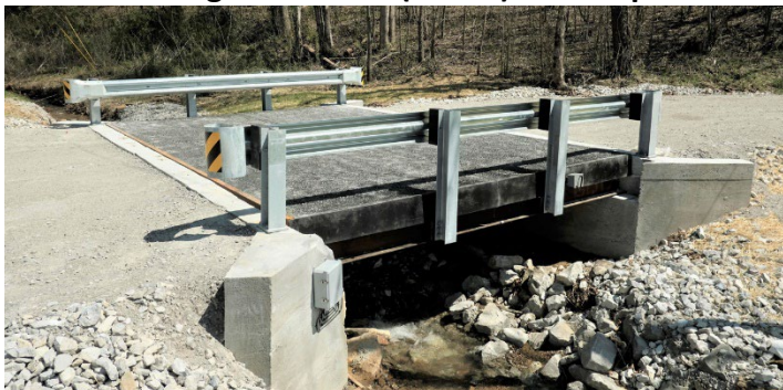
Figure 8: First fiber-reinforced polymer vehicle bridge deck in Tennessee Credit: IACMI
